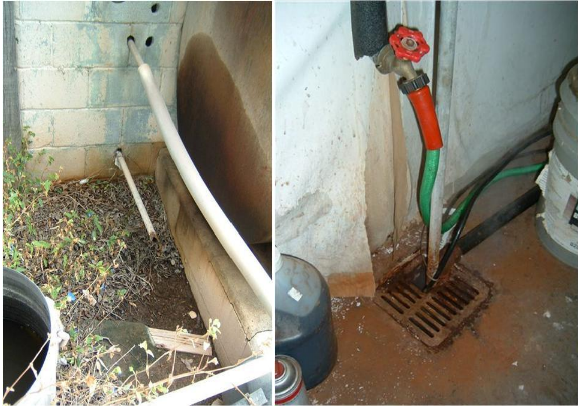
Discharge points: To bare ground (left photo) and to floor drain to sewer (right photo)
