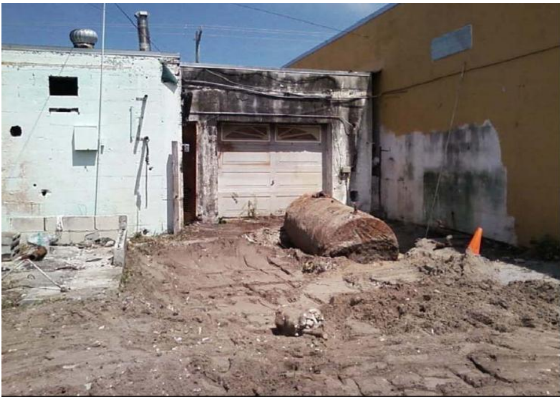
Solvent Product UST at Rear of Dry Cleaner
