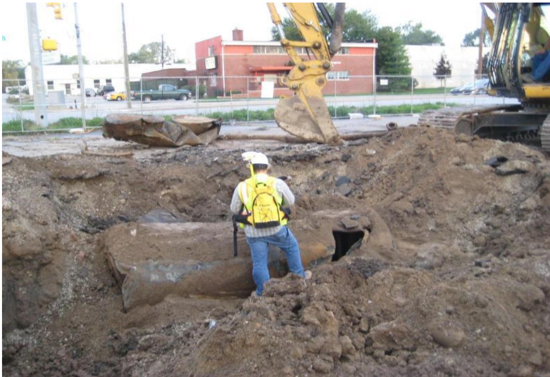
Dry Cleaner Solvent Product UST Removal
